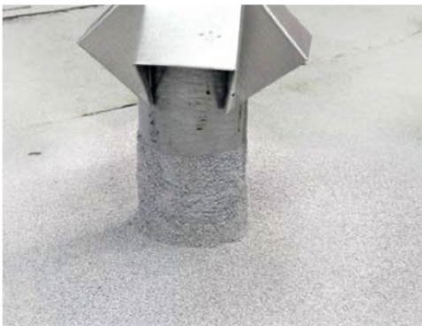
Fig. 7a: Embed matching granules in Ply-Flash Compound
