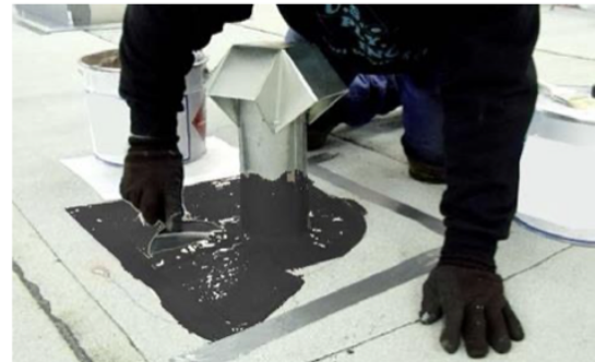
Fig. 4 Spread Ply-Flash Compound with trowel or spatula.
