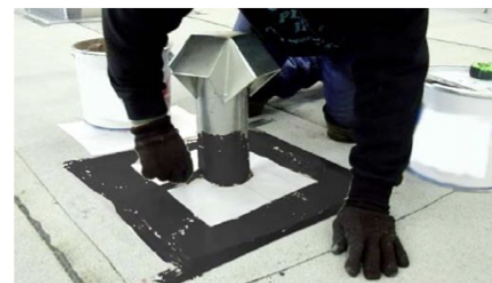
Fig. 5: Embed reinforcement in Ply-Flash Compound
