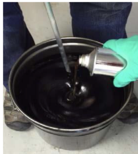
Fig. 2 Pour Part B (hardener) into Part A (modified asphalt) while stirring Part A. Strictly follow mixing times to achieve proper mix.
