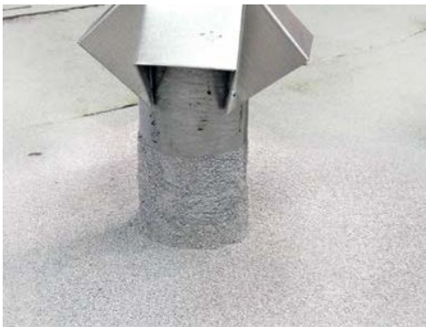
Fig. 7a: Embed matching granules in Ply-Flash Compound
