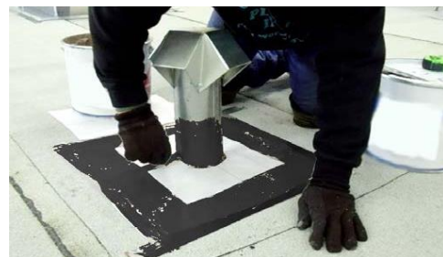
Fig. 5: Embed reinforcement in Ply-Flash Compound
