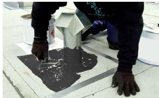
Fig. 4 Spread Ply-Flash Compound with trowel or spatula.
